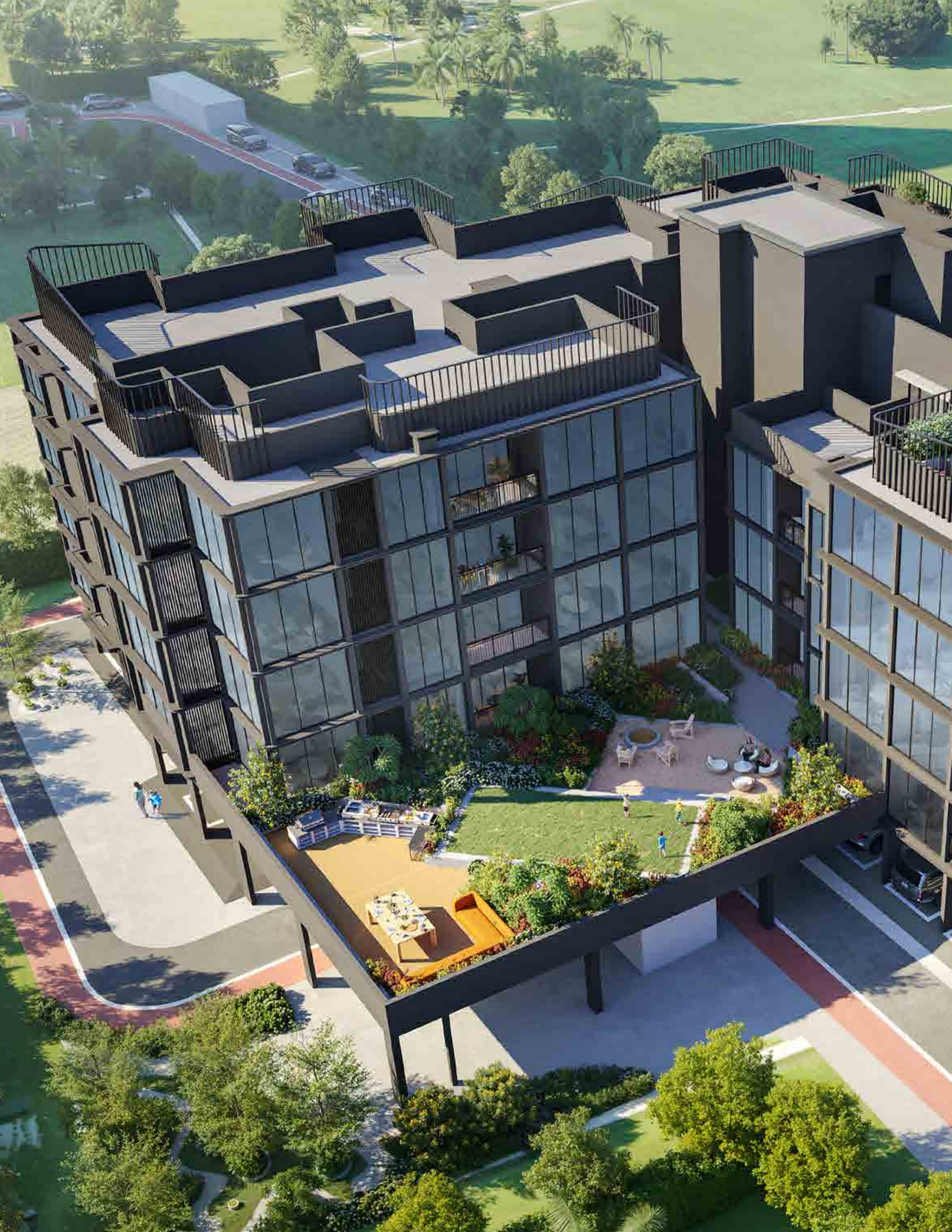
ELEVATION AERIAL VIEW
